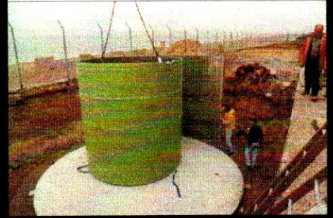
9. After the outer sill has been formed and the concrete has cured the Camplas Fiberloc Tank is ready for use.
