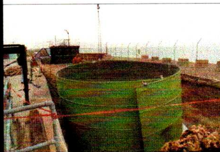
7. Almost completely un-rolled and nearly in place the tank is starting to take shape.
