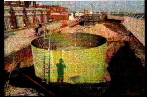
9. After the outer sill has been formed and the concrete has cured the Camplas Fiberloc Tank is ready for use.
