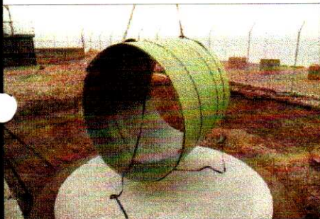
7. Almost completely un-rolled and nearly in place the tank is starting to take shape.
