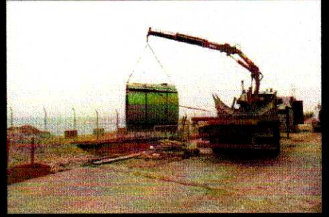
6. The tank is now ready to be un-rolled by the workmen so that it fits around the foundation.
